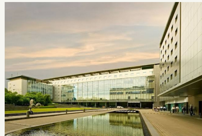
Panchshil Tech Park One, Yerwada Five towers on Airport Road. Corporate services and managed ops find it practical.
