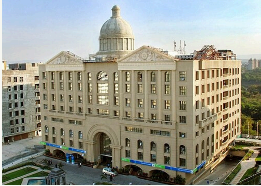
Cerebrum IT Park (Kalyani Nagar): Situated near the city center, this park houses companies like Capgemini and Tech Mahindra.
