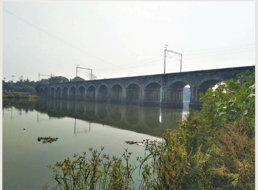
DAPOORIE RAILWAY BRIDGE AS OF NOW
